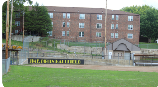
Jim E Piburn Ballfield Amenities: 1 baseball/ softball field, basketball and playground
